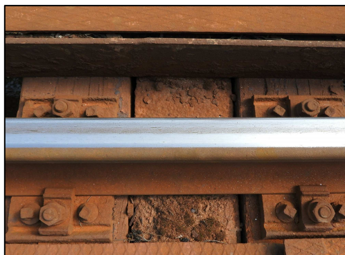
obr. 24: svršek K 01, podkladnice
